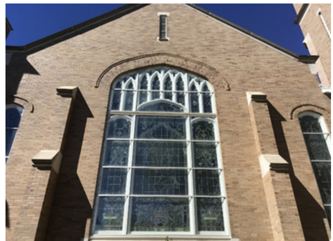
Stained glass window repair, Pierre Methodist Church
